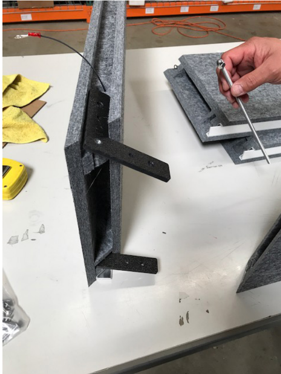
1) Place L brackets(2) into the Airebaffle™ using designated brackets(TOP, BTM) keeping markings facing up.
