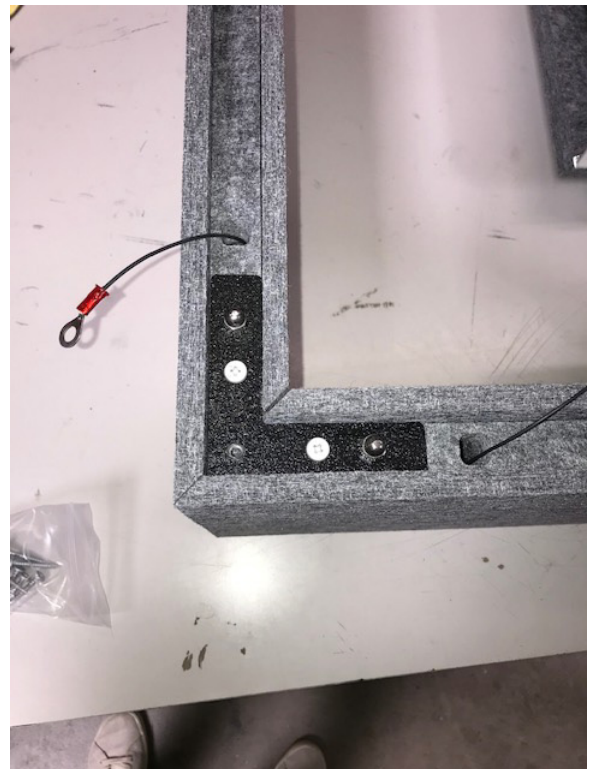
4) Insert safety screws(2) into center holes of L bracket.
